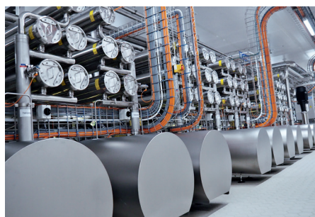
A RO process requires substantial pressure that is built by a row of heavy pump equipment by Alfa Laval (photo: IDM)
